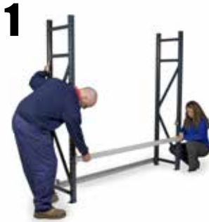
1 Position a pair of frames. Hold them in place with a pair of beams
